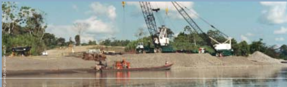
Cranes digging vast quantities of construction materials from the Unubamba river bank along the right of way for the Camisea gas pipeline in Peru, August, 2002
