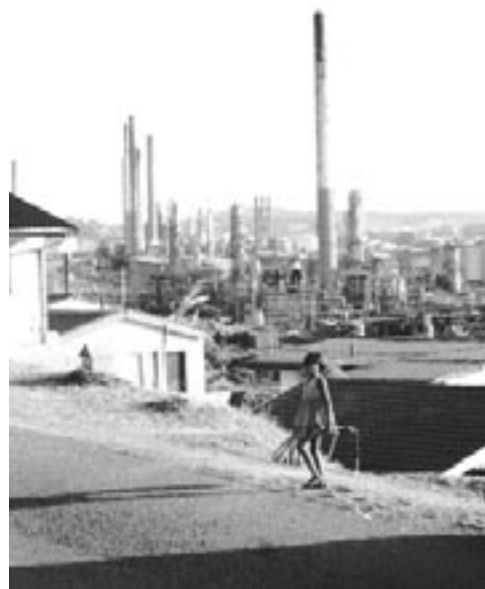
The South African Petroleum Refinery (SAPREF) in south Durban.
